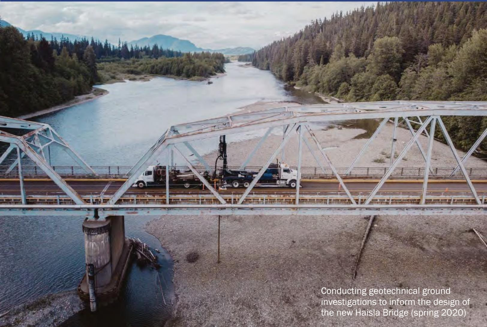
Conducting geotechnical ground investigations to inform the design of the new Haisla Bridge (spring 2020)
