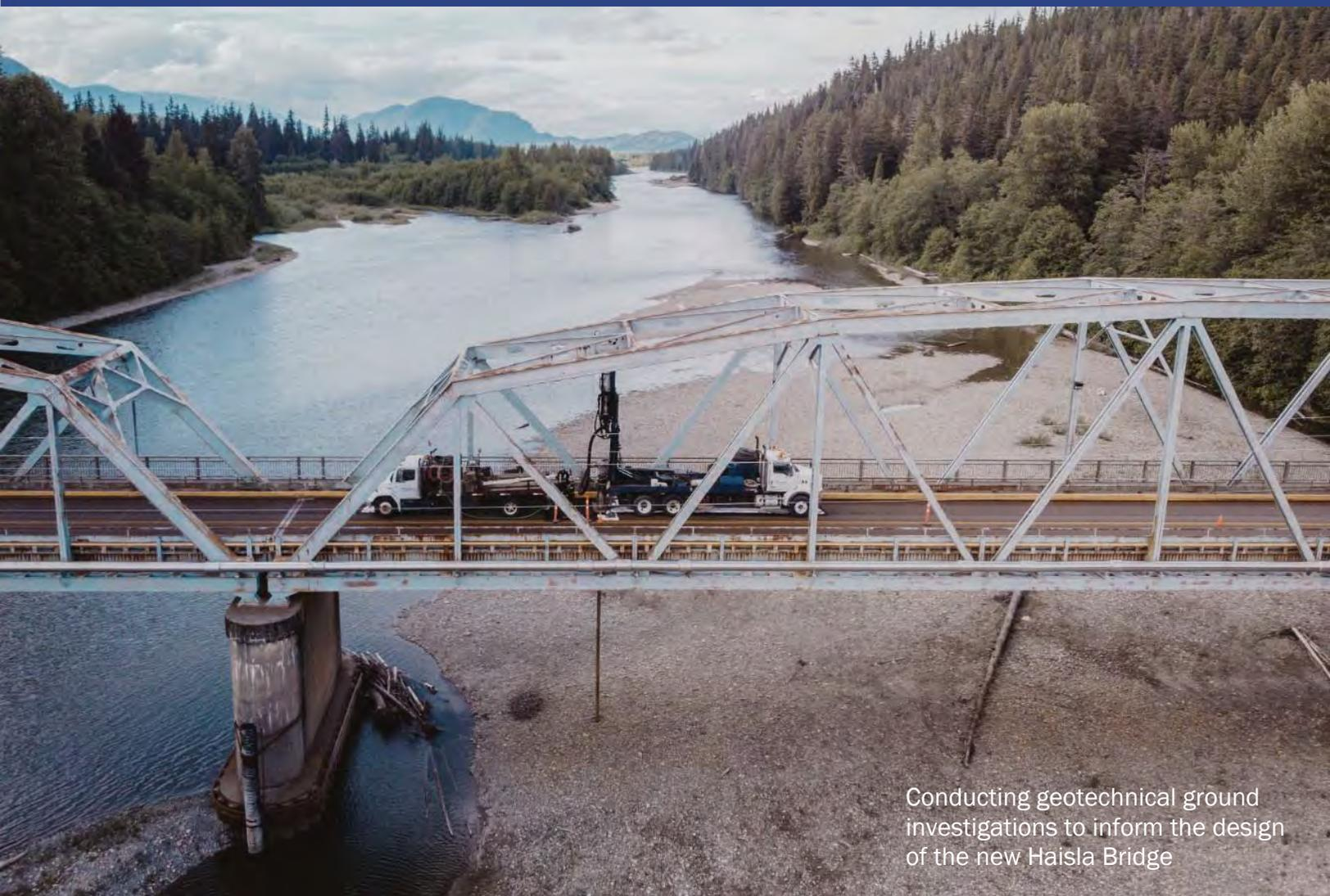
Conducting geotechnical ground investigations to inform the design of the new Haisla Bridge
